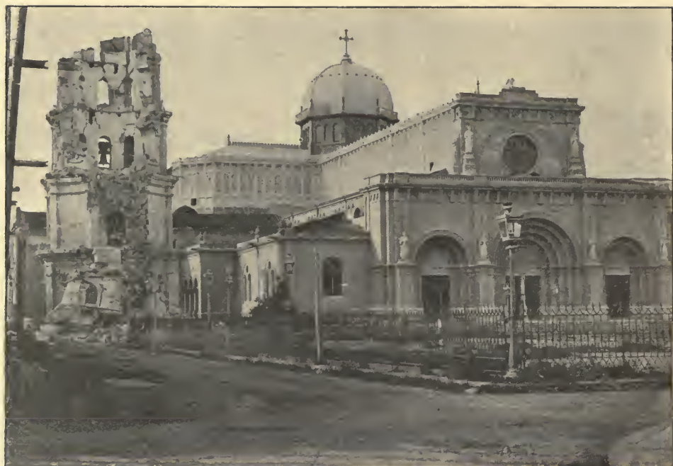
CATHEDRAL OF MANILA AFTER EARTHQUAKE.
